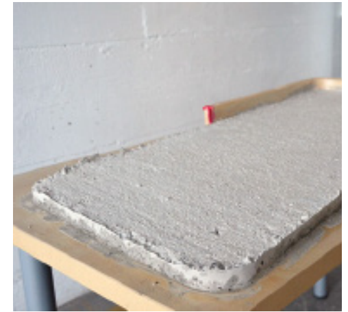
Fig. 70. Coffee Table Process 6. With half of the PELLO mold removed, the corners of the concrete top can begin to be gently pried up. (Photograph by M. Harkness, 2016)
