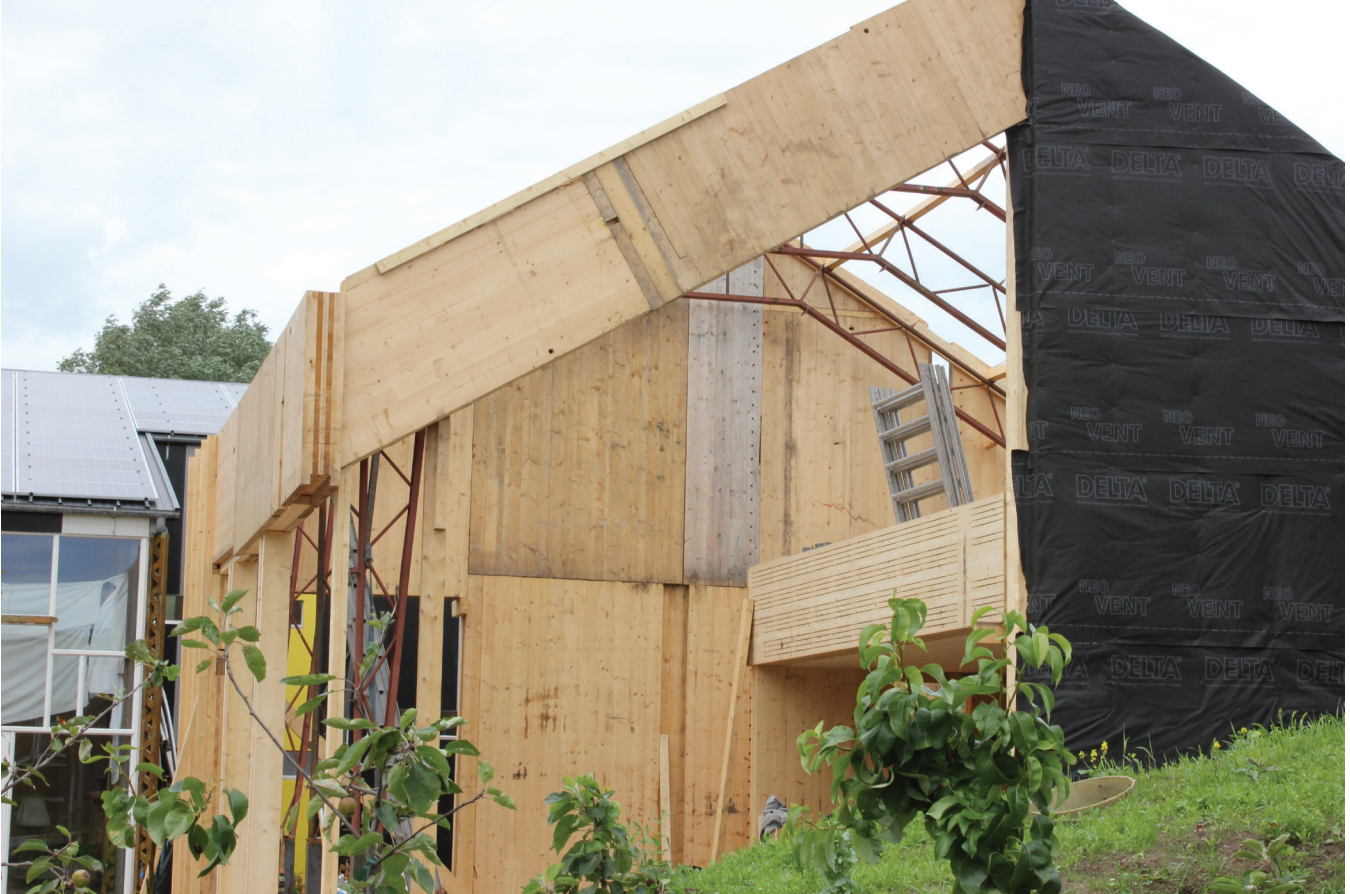
Fig. 46- This new workshop and material repository building was under construction at the time of my visit. Materials were sourced from a development site in The Hague. The laminate wood had been cut incorrectly for the construction plans.
